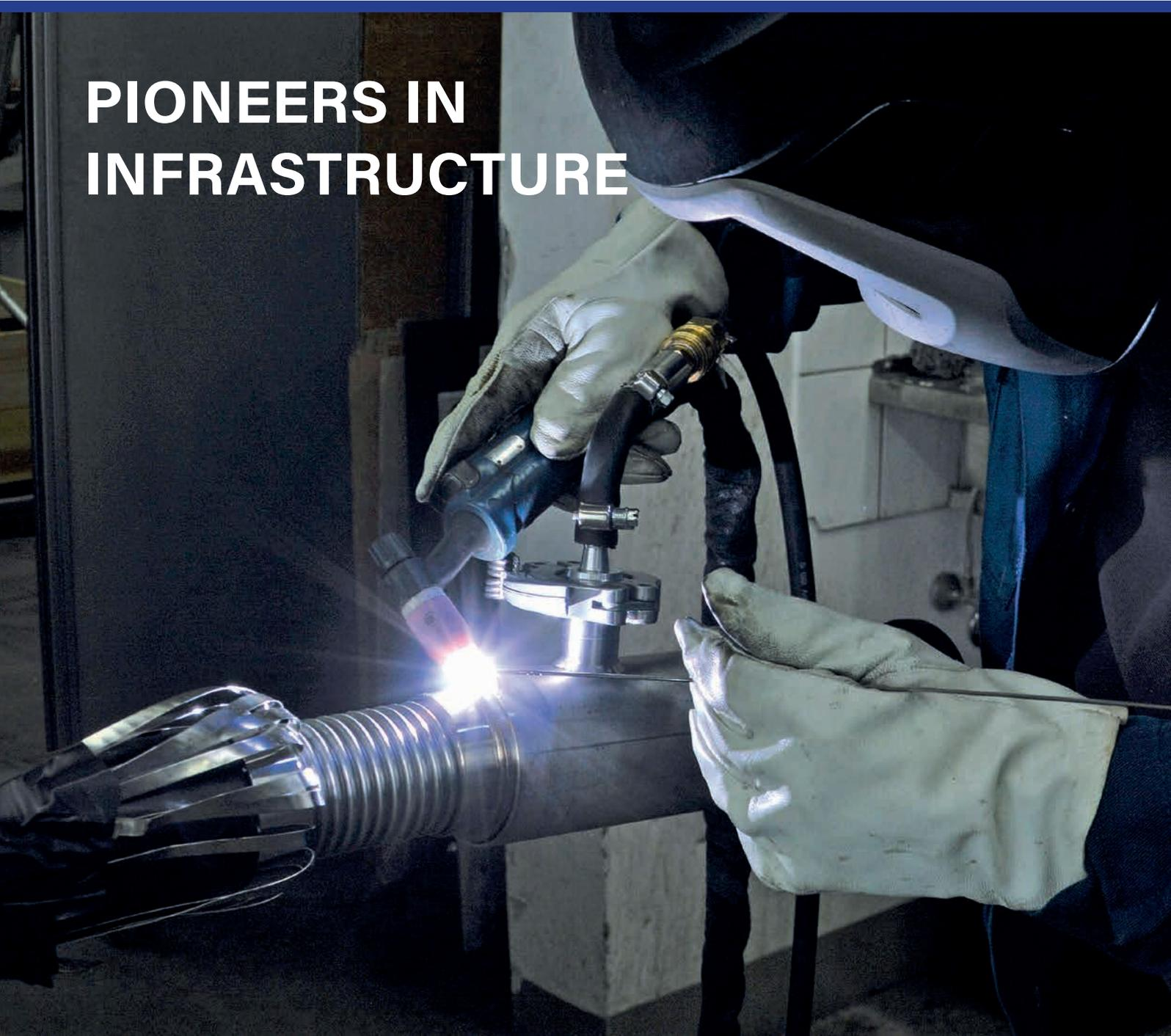
A close-up photograph of a welder wearing a dark protective suit and a white face mask. The welder is using a welding torch to join a metal pipe. The pipe has a corrugated section on the left. A bright light from the welding process is visible at the point of contact. The background is dark and industrial.
