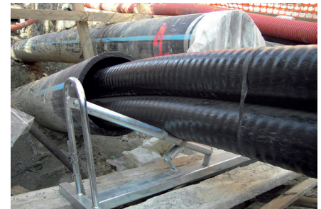
The pipes before inserted into the PE-HD jacket pipe
