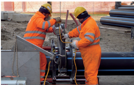
Welding of the jacket pipes
