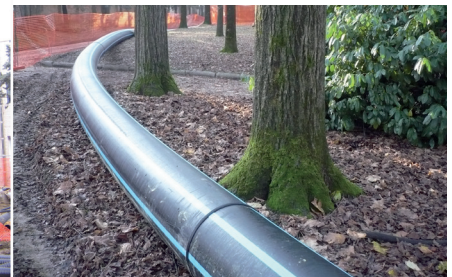
Ready for trenchless laying
